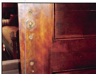
The interior side of the front door after re-drilling.
