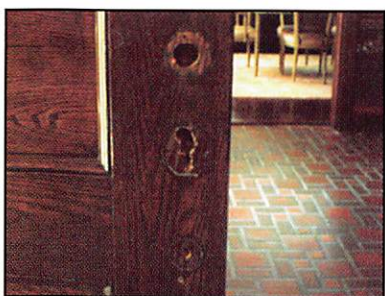
A view of the exterior of the door with the existing hardware removed and a bit of re-drilling.
