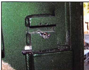
Photo 12 has the two Allen head cap screws backed out to allow the cylinder to come out.
