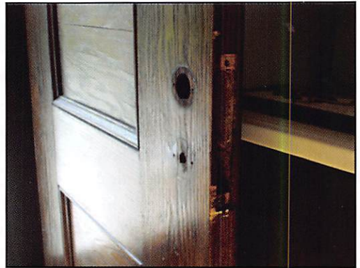
The rear door with the old Reading lock removed.
