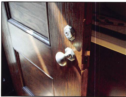
The rear door before we started. Note that the cylinder is off center, since the set screw that should hold it in place is missing.
