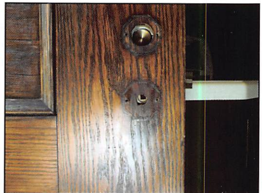
The old removed, and the new mortise case installed in the door. Note that the holes match up pretty closely!
